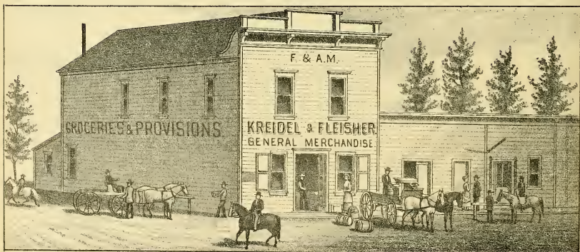
STORE & AGENCY OF WELLS FARGO & CO'S EXPRESS, KREIDEL & FLEISHER, CENTRAL CITY, STA MARIA VALLEY, SANTA BARBARA CO. CAL.
